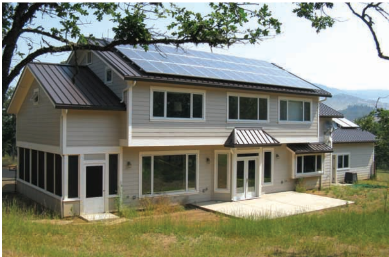
Southside provides passive solar access. PV and solar hot water on rooftops. No southside roof penetrations to interfere with solar devices. Credit: Karen Chase, Oregon Dept. of Energy
